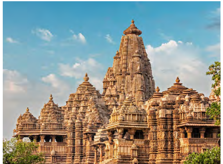
Image 2. 10: Domed Roof at Khajuraho Temple, Madhya Pradesh
