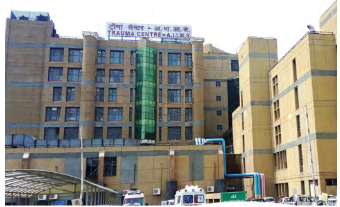
Image 4. 2: Jai Prakash Narayan Apex Trauma Centre at AIIMS Delhi uses Trigeneration System
