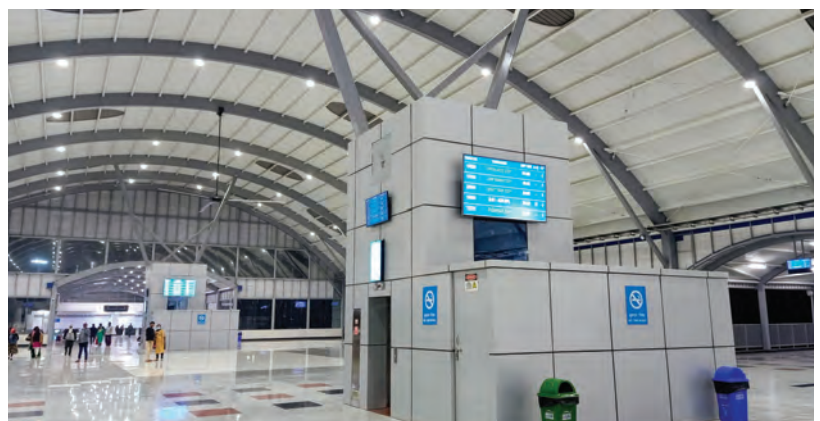
Image 3. 3: Rani Kamlapati Railway Station, Bhopal
